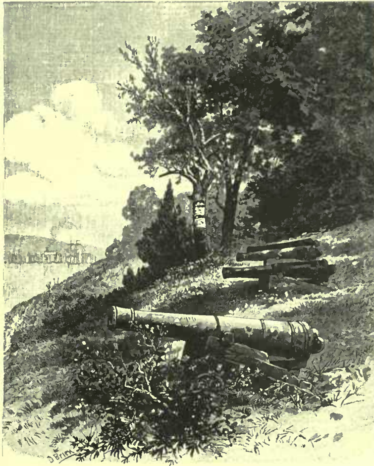
OLD BATTERY, ST. HELEN'S ISLAND.
